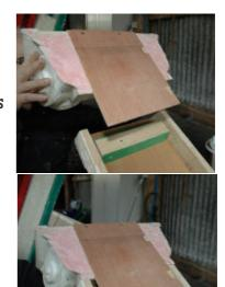
Stand columns in place & secure with final fixing screw
