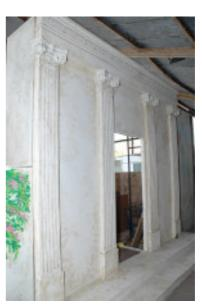
Screw the terrace backing S18 to the back of S2 & S3 by screwing through the steel frames. Then fix the columns & column tops with one screw to the backing
