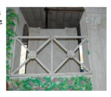
Finally screw the rail in place (through the steel frames) & fix doors. 2 door closers are provided.
