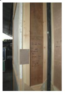
Attach flat S16 using ply plates.
