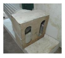
Place the columns upright with the bolts locating in the holes in the step.
