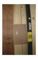
Ply plates & screws are used to join flats together. The plates should be already screwed to one flat. Just butt the flats together & fix with 2 screws as shown. When striking set, only remove the 2 screws you have put in & leave plate attached the the original flat. Do not remove screws that have a  $\bigotimes$
