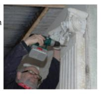
When all 4 columns are fixed, the pediment should be put into place & secured. There are 4 blocks of wood in the back of the pediment to take wood screws driven in from the back of the flats. Care should be taken when fixing pediment to avoid damage to the fragile column tops.
